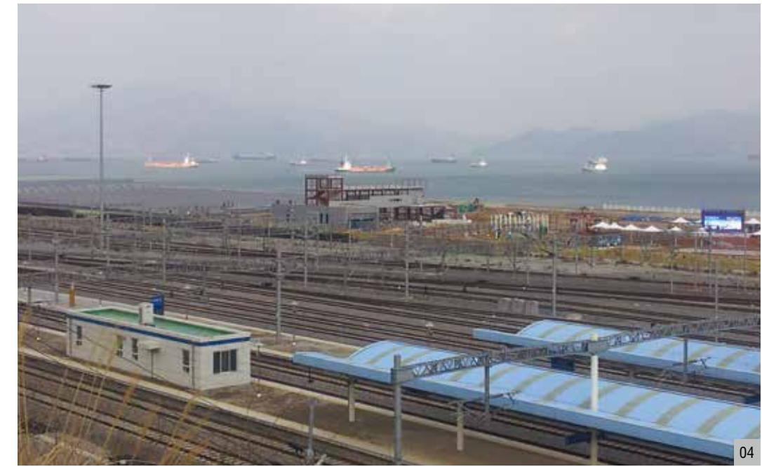
04 Railway power facility of the Suncheon – Yeosu section in the Jeolla Line (Jeonnam, Korea) • Completion : 2012.05
