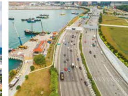
Marina Coastal Expressway, Singapore
