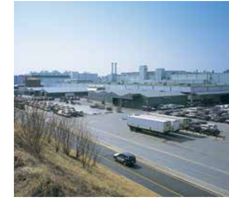
04 Ssangyong Motor Co. Plant (Gyeonggi, Korea) • Completion : 1991.12
