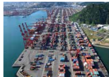
Busan Port Shinsundae Container Terminal
