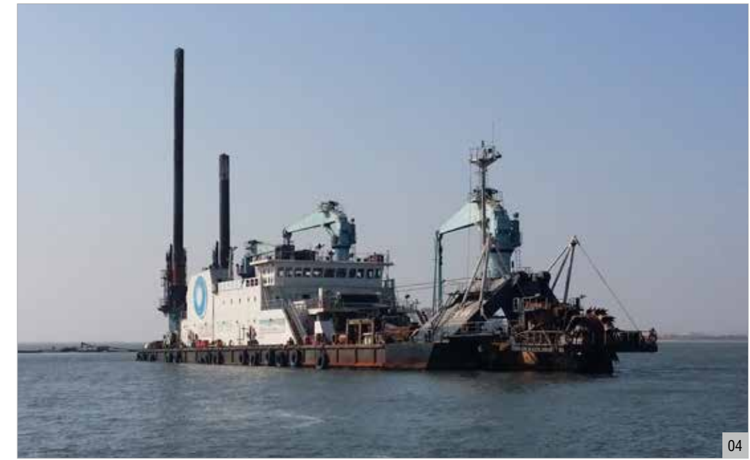
04 Gunjang Port Sea Route Dredging Project - Stage 2 (Gunsan, Korea) • Completion : 2019.12
