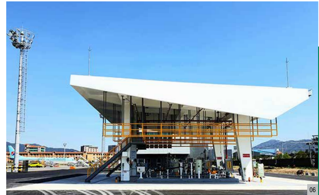
06 Gimhae Airport Aircraft Oil & Gas Storage Tank (Busan, Korea) • Completion : 2019.04 • Client : Korea Airports Corporation • Three underground aircraft oil & gas storage tanks (13,000 bbl), hydrant facilities
