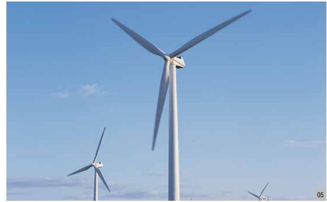
05 Wind Power Plant, Jeju Island (Jeju, Korea) • Completion : 2000.01
