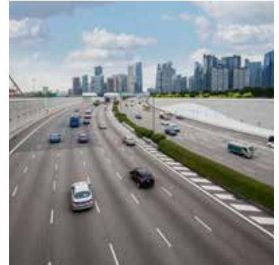
Marina Coastal Expressway (Singapore)
