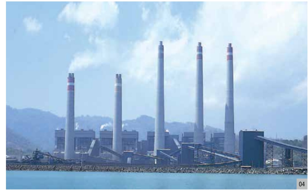
04 Suralaya Steam Power Plant (Indonesia) • Completion : 1996.06 / Client : Perusahaan Umum Listrik Negara(PLN)
