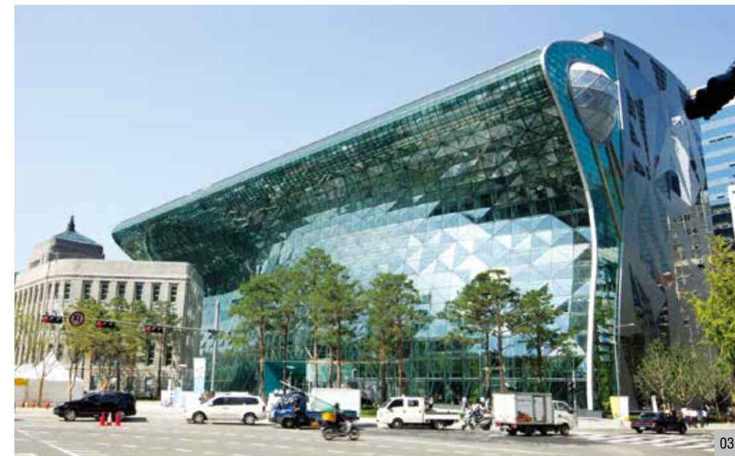
03 Seoul Metropolitan Government Building (Seoul, Korea) • Completion : 2012.08 • G-SEED certified in 2013 • Application of new and renewable energies (geothermal heat, solar heat, solar energy, natural lighting)
