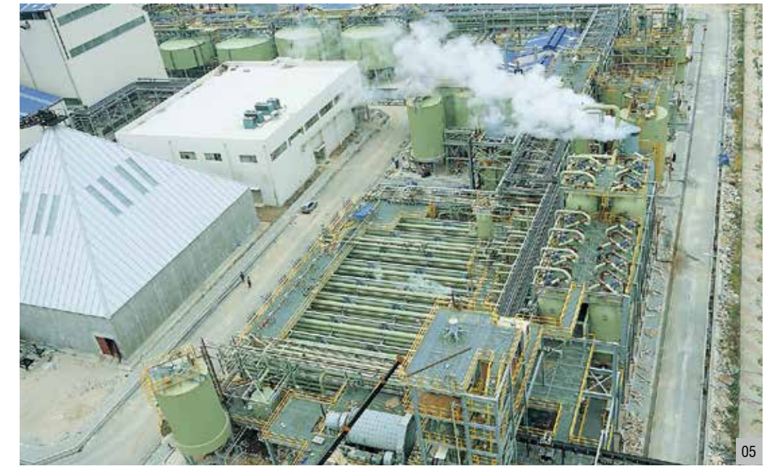
05 Aluminium Hydroxide Production Plant (Jeonnam, Korea) • Completion : 1995.11
