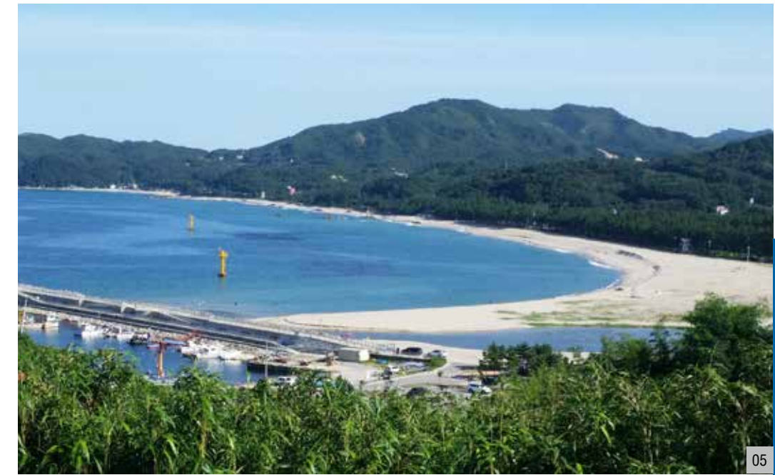
05 Gungchon Port Erosion-Sediment Reduction Facility Construction Project (Samcheok, Korea) • Completion : 2016.11
